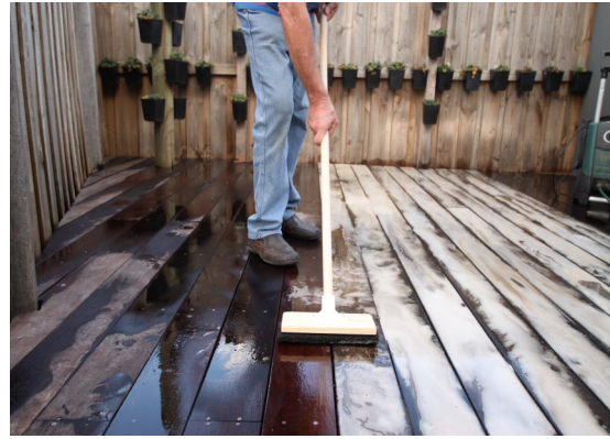
Cleaning Merbau decking
