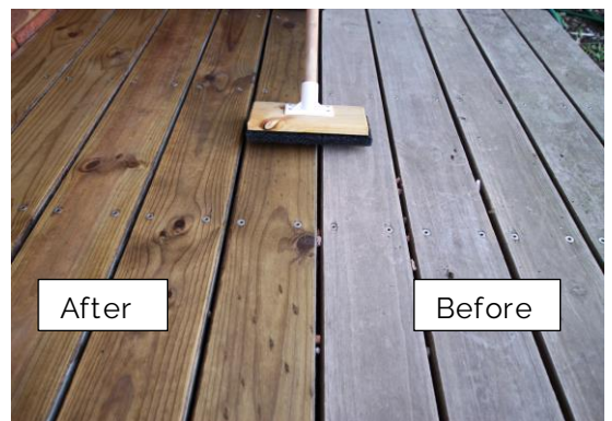
Cleaning & Oiling Treated Pine Decking
