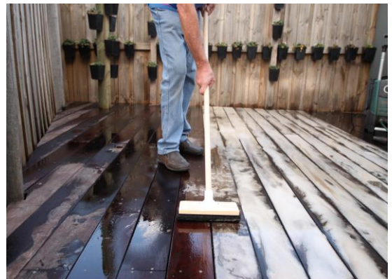
Cleaning Merbau Decking
